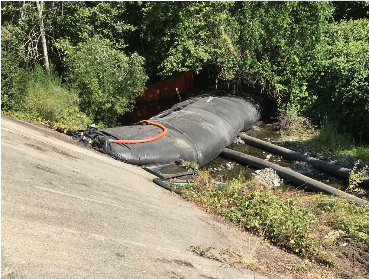
Upstream Coffer Dam in Creek
