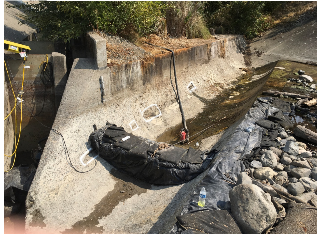
Upstream Coffer Dam in Sediment Trench
