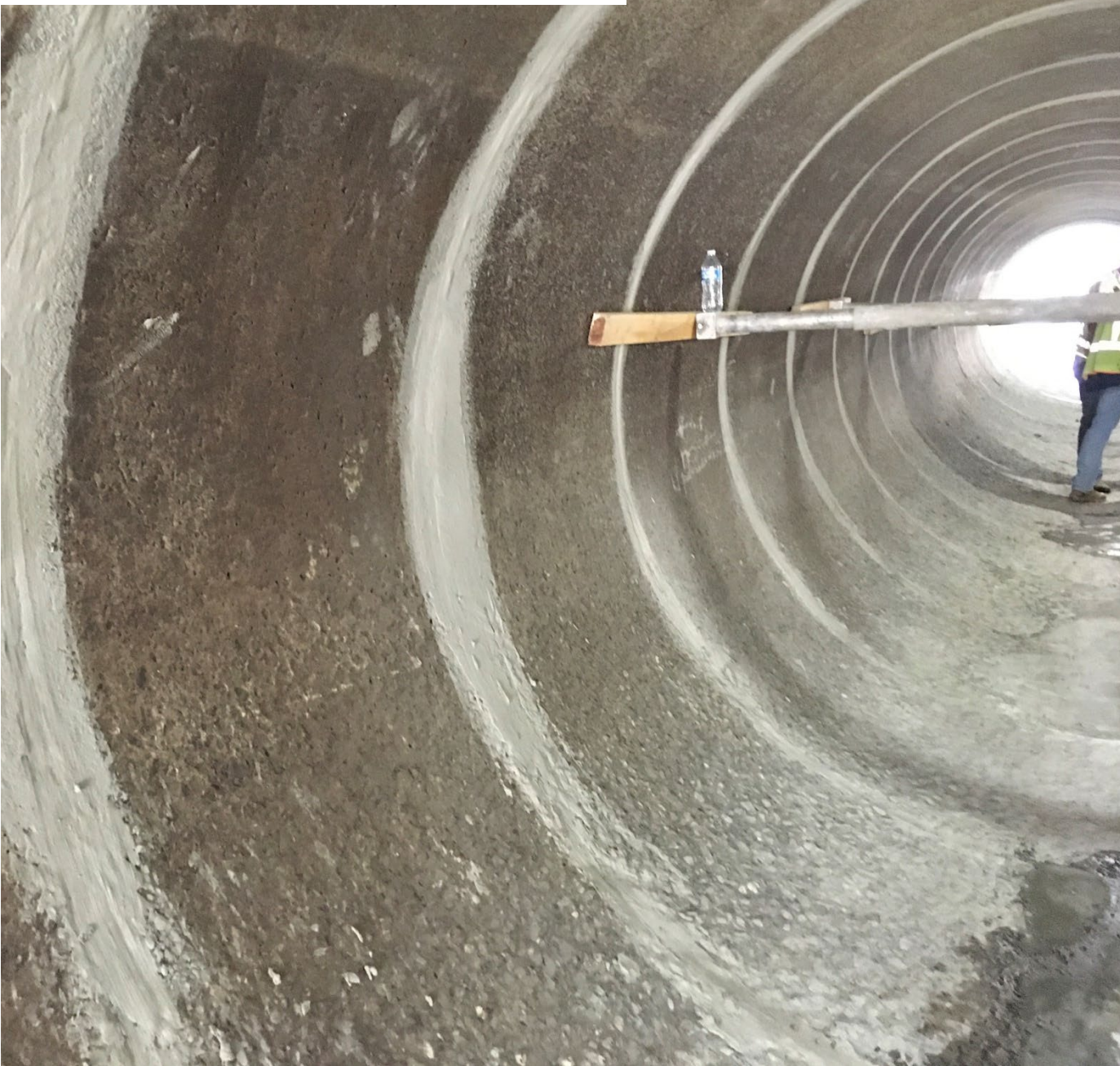
Repaired seams prior to FRM
